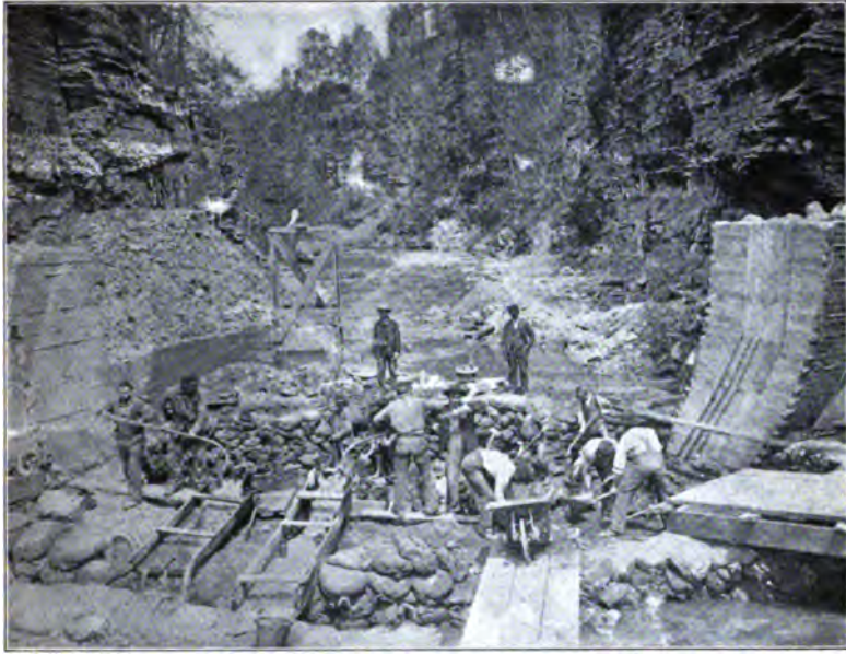
FIG. 1.—PREPARING THE FOUNDATIONS FOR THE SIX-MILE CREEK DAM.
